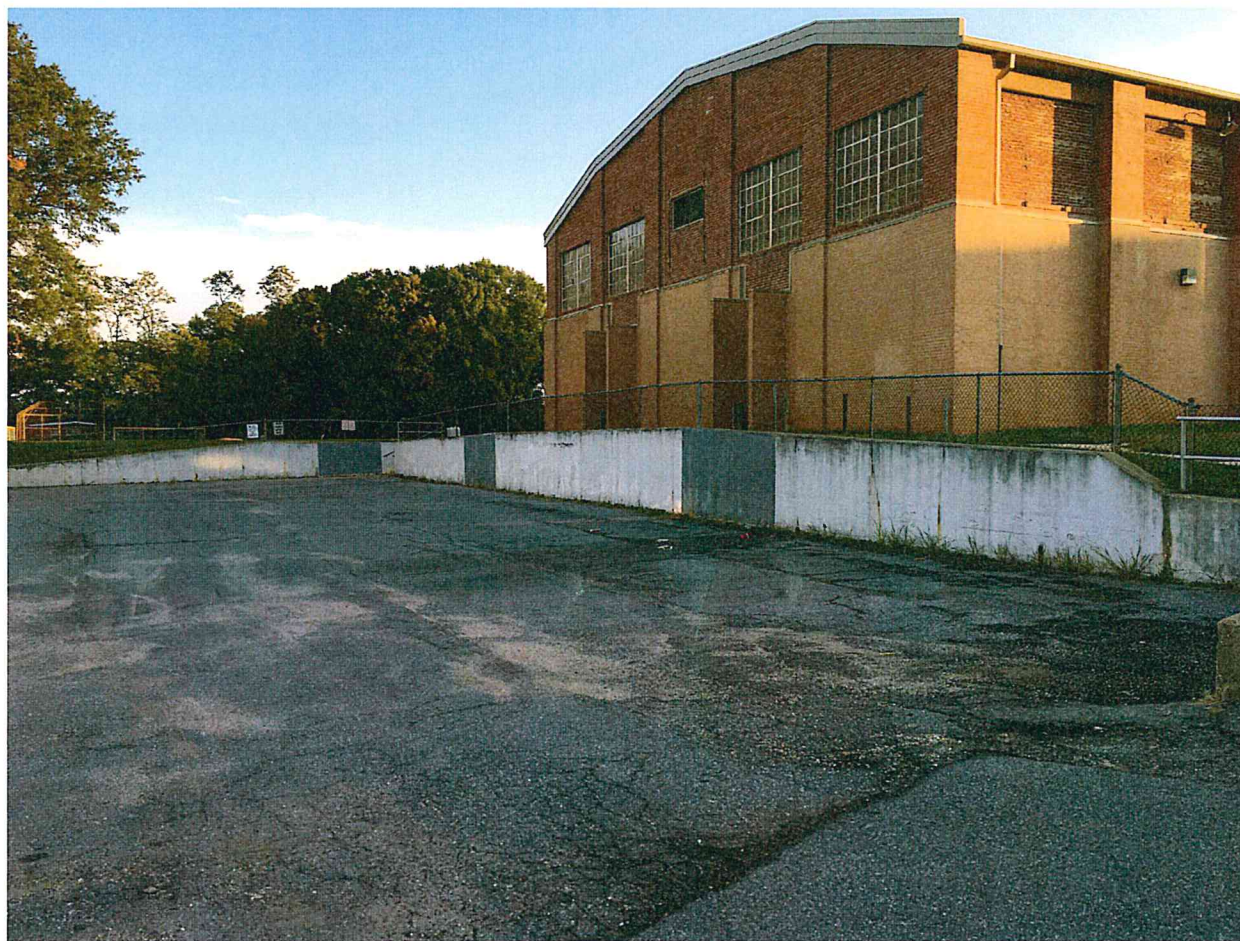
Exhibit 1: HMS Exterior Retaining Wall
