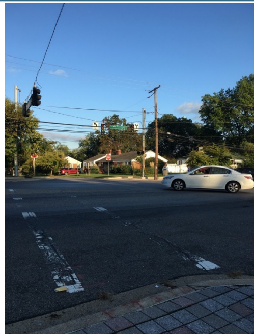
Figure 17: Missing Curb Ramps in Front of St. Jerome Academy (left); Faded Crosswalk on Adelphi Road (right)
