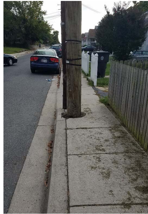
Figure 11: Existing Sidewalk Obstruction on Local Street
