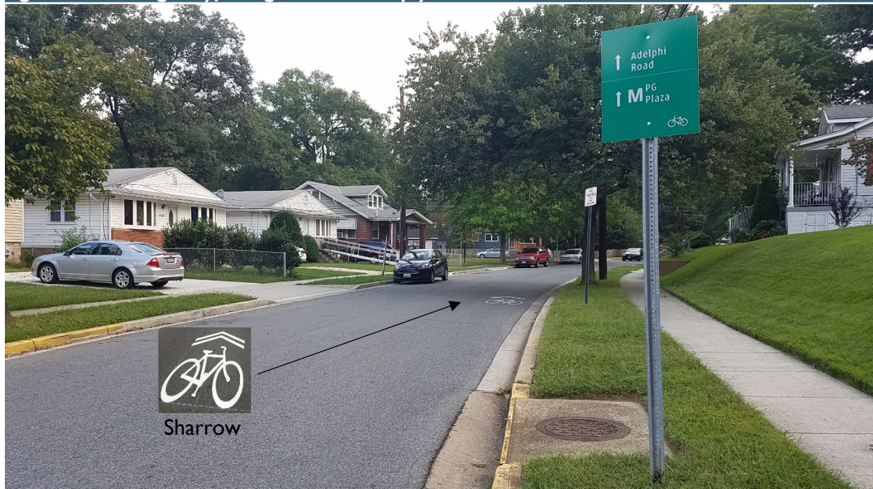
Figure 20: Existing Wayfinding does not comply with current MUTCD Standards
