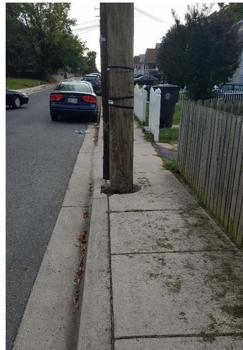
Figure 11: Existing Sidewalk Obstruction on Local Street
