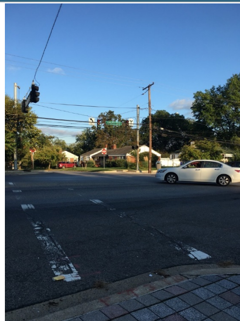
Figure 17: Missing Curb Ramps in Front of St. Jerome Academy (left); Faded Crosswalk on Adelphi Road (right)
