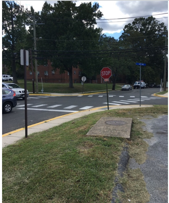
Figure 6: Existing High Visibility Crosswalk on Intersection of Oglethorpe Street and 42 nd Avenue
