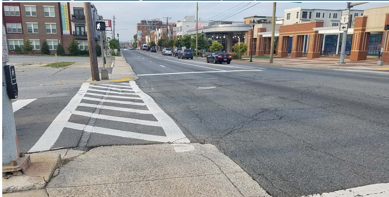
Figure 16: Existing conditions along Baltimore Avenue (Route 1)
