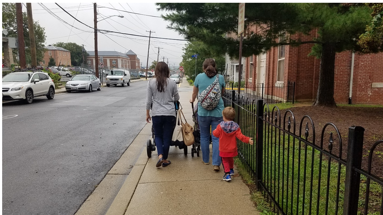
Figure 19: Existing Sidewalk is too Narrow to Accommodate side-by-side stroller traffic.
