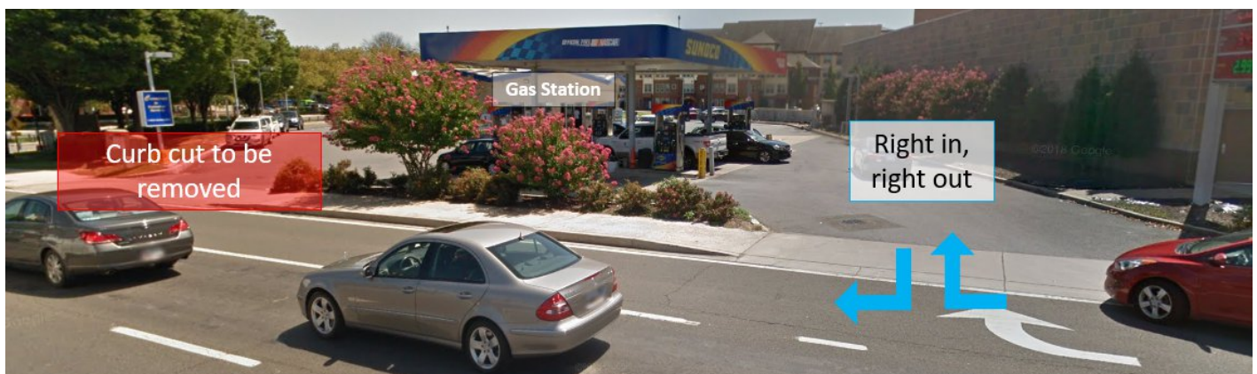
Above: View of Site from East-West Highway. Curb cut to be removed as indicated in DSP-19039 and proposed remaining curb cut are depicted.
