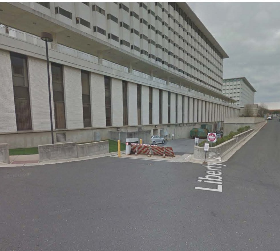
NORTH FACADE | ENTRY TO LOWER LEVEL PARKING
