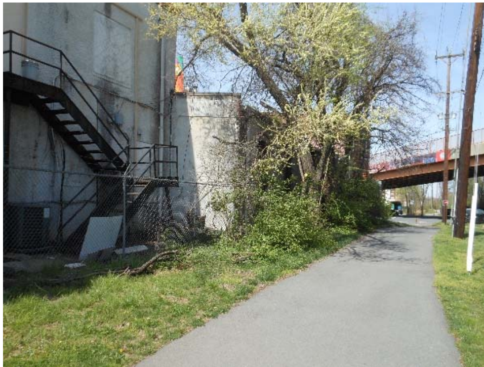
Figure 19 - Northbound view near the Trail Head in Hyattsville, MD. Area needs removal and maintenance of overgrown vegetation.
