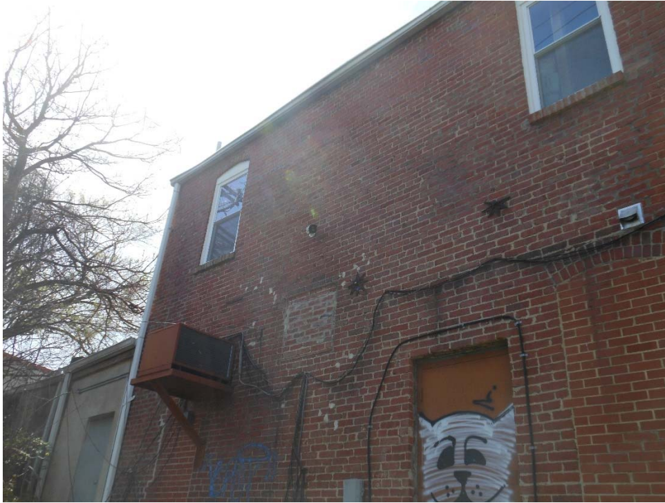
Figure 20 - View of graffiti on the back of one of the commercial buildings near the Trail Head in Hyattsville, MD. Potential location where brick could be painted a light or bright color to enhance brightness of the area.
