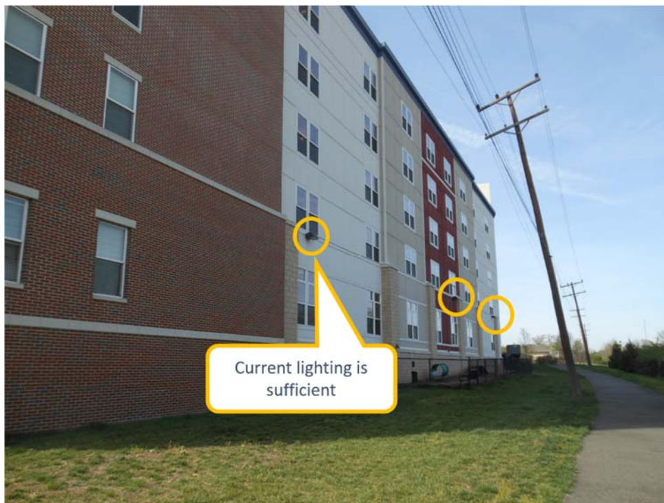
Figure 8 – Lighting installed behind the Palette Apartments & Townhomes in Hyattsville provide sufficient illumination for this segment of the Trail.
