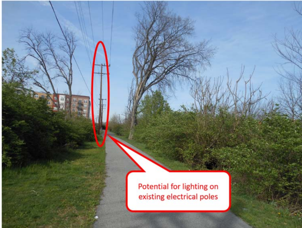
Figure 4 - Northbound view from the Baltimore Avenue overpass in Hyattsville, MD. Existing utility poles located along the Trail could be utilized to install lighting.
