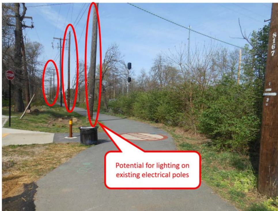
Figure 6 - Northbound view near the Madison Street Trail access point. Existing utility poles located along the Trail could be utilized to install lighting.
