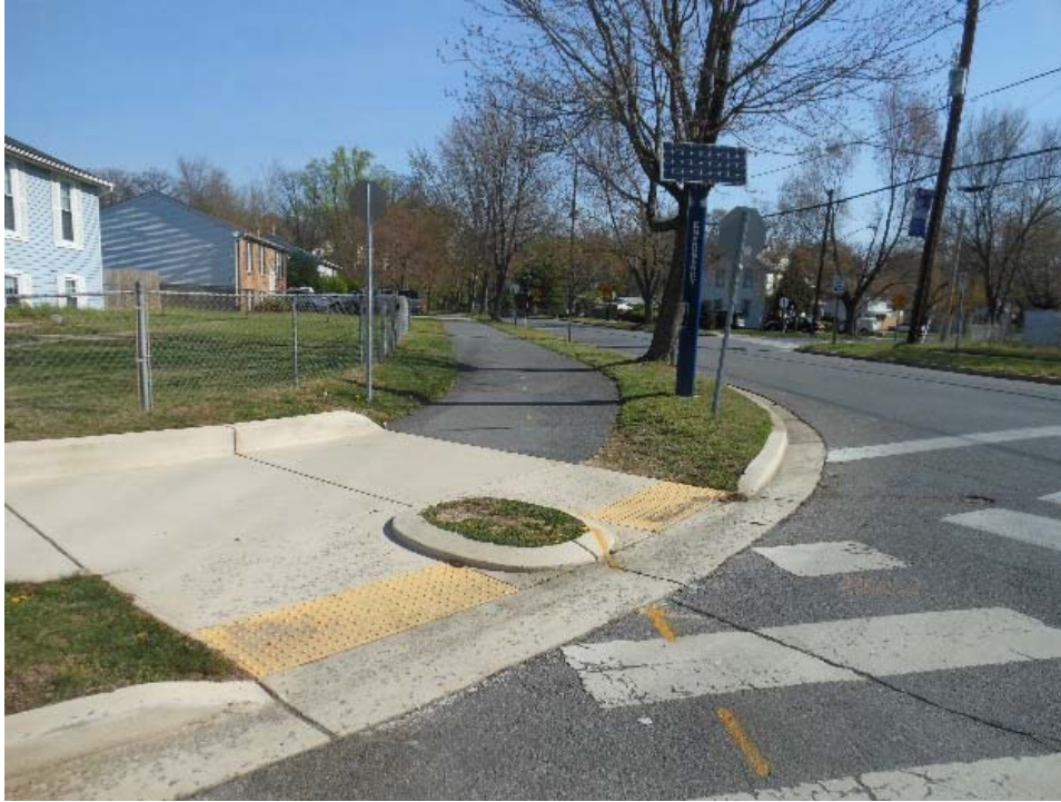
Figure 36 - Typical raised symbolic barrier used in the College Park area of the Trail. Note the low-profile design, which would not stop a motor vehicle from passing over it.
