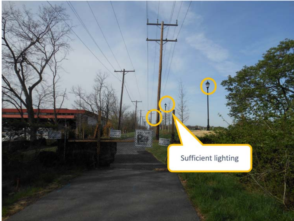
Figure 14 – Northbound view from the southern end of the Cafritz development temporary closure. Newly installed lighting at the development will sufficiently illuminate this section of the Trail.
