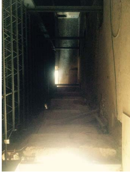
View of back from existing stair wall
