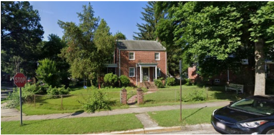
Figure 1: Street View from Madison St.
