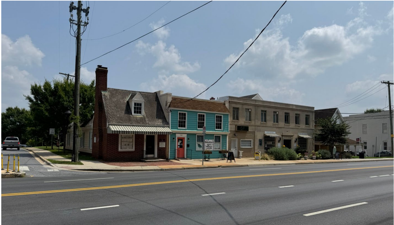
Figure 3: 5301-5309 Baltimore Avenue, existing conditions, from north.
