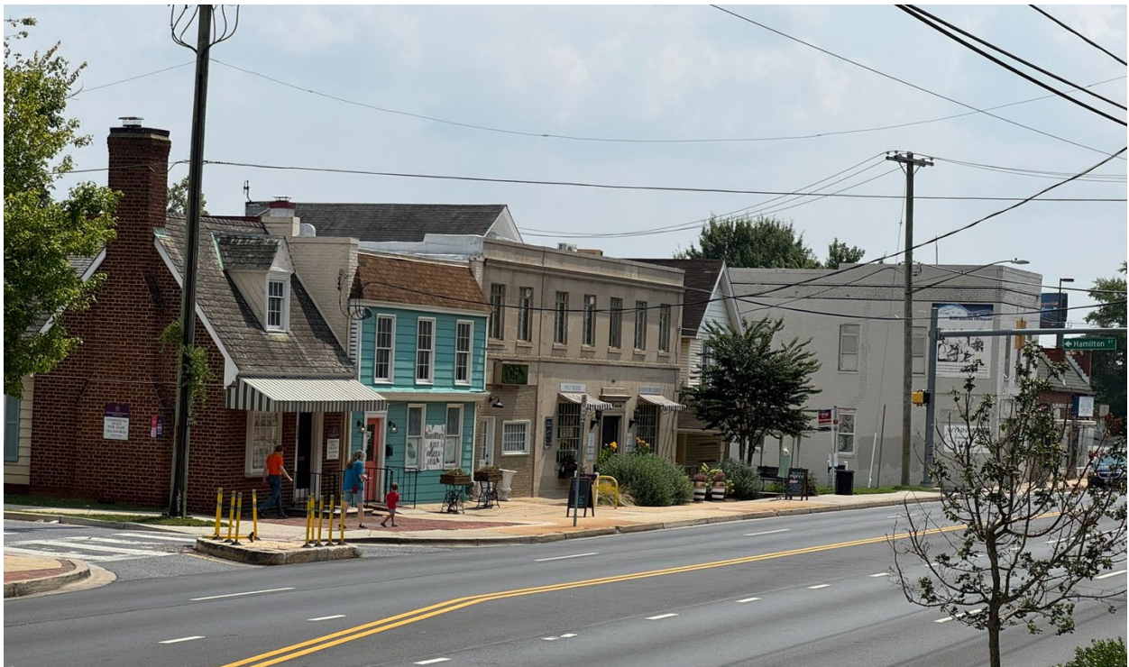
Figure 4: 5219-5309 Baltimore Avenue, existing conditions, from north.
