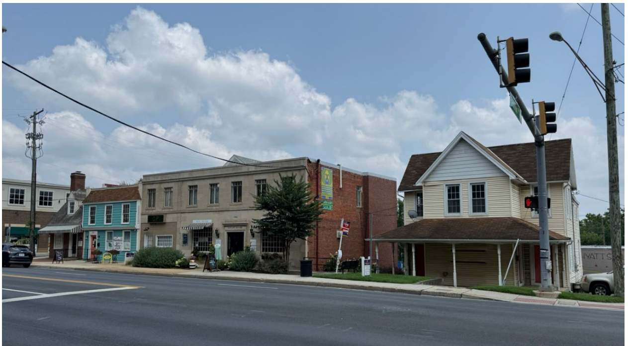
Figure 2: 5301-5309 Baltimore Avenue, existing conditions, from south.
