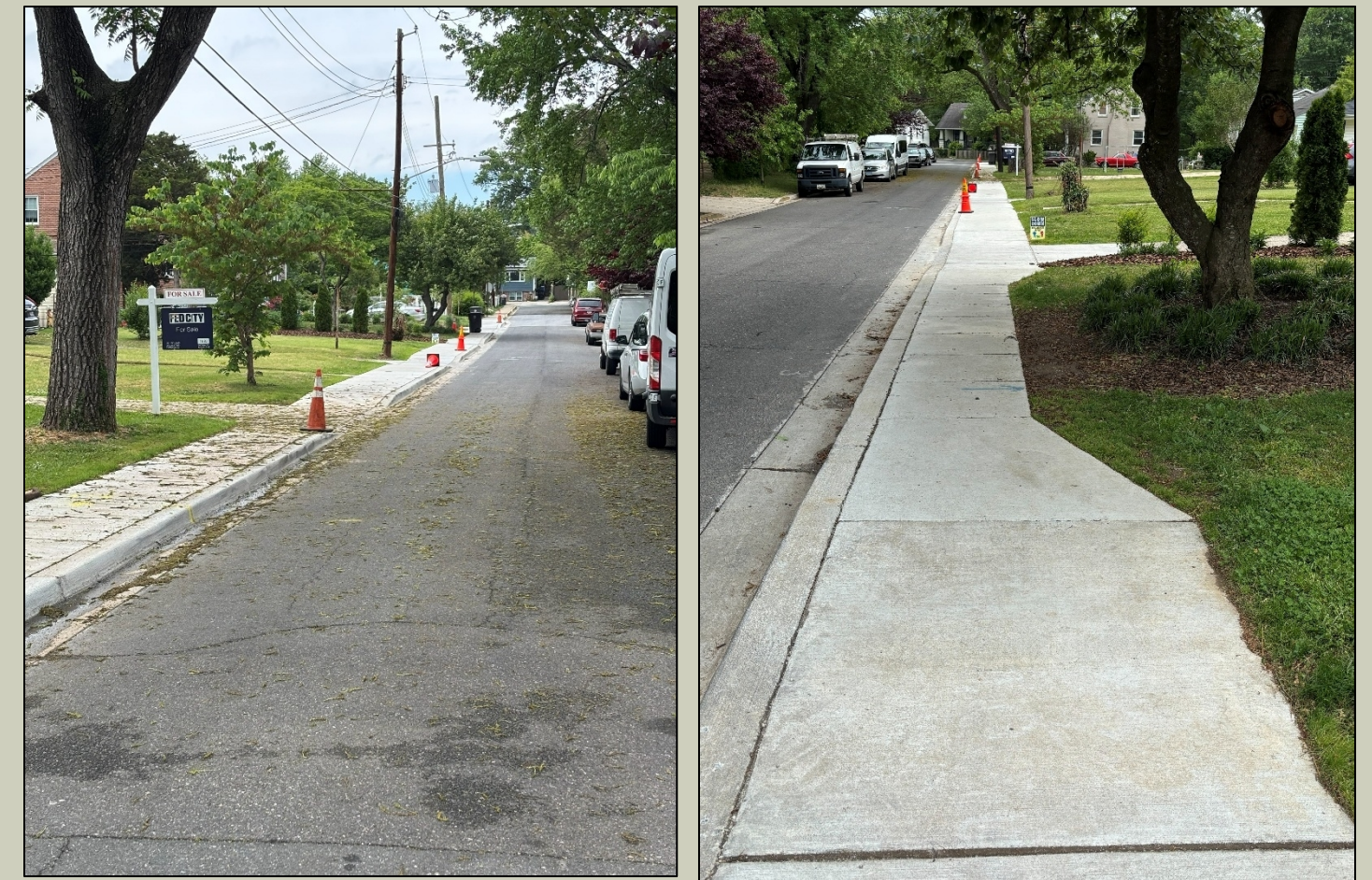
Installed sidewalk, spring 2026
